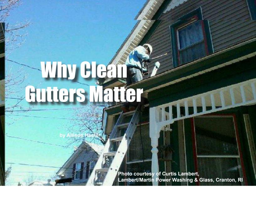
affordable methods for homeowners to protect their homes from the elements. By channeling water off the roof and directing it to a location away from the home, properly working gutters help protect the home's shingles, wood under the eaves, siding, flooring and landscaping from a whole host of problems and expensive repairs. These include:
