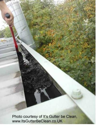
questions, the general rule of thumb is that most gutters should be cleaned twice a year. Fall and Spring are usually the months of choice because that is when they gutters become the most clogged due to falling leaves, pine needles, blooms, seed pods, and so on.
